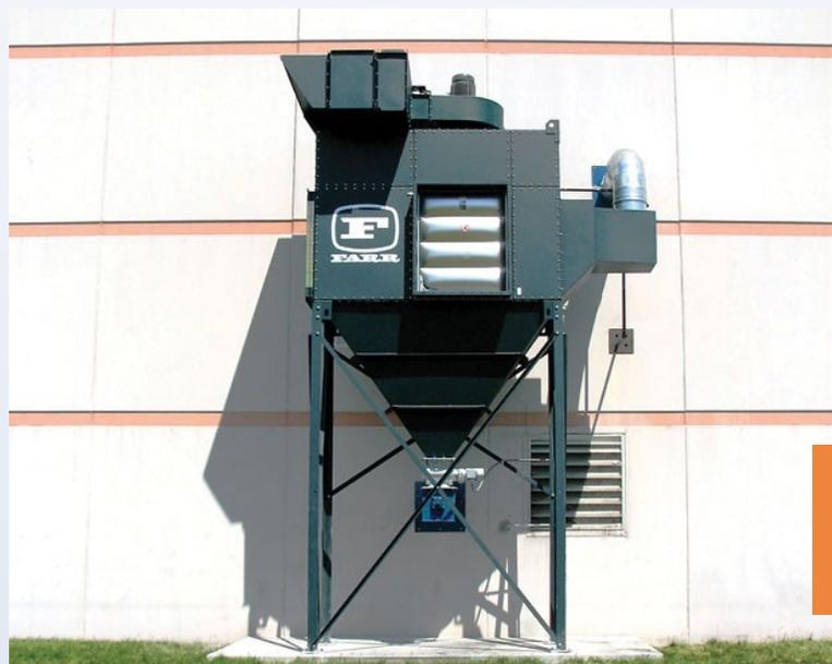
This dust collector is equipped with an explosion vent with vertical upblast deflector plate. *Photo Courtesy of Camfil APC*
